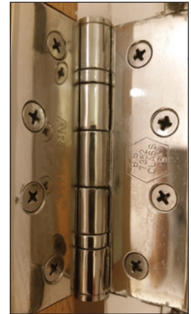
Compliant hinges on older doors were tested to BS 7352; class 8 for a 30 minute door and class 9 for 60 minutes.
